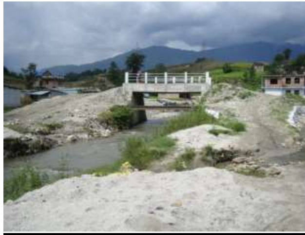
Dhobikhola Corridor Bridge (Completed)
