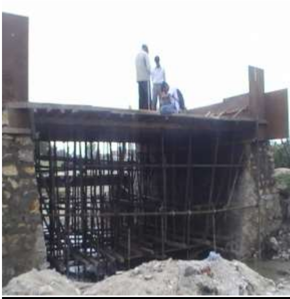
Dhobikhola Corridor Bridge at Chunikhel
